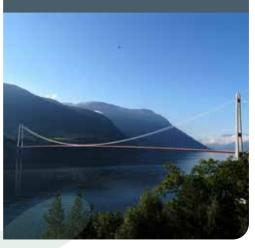
THE HARDANGER BRIDGE opened on August 17th 2013, replacing the ferry connection between Bruravik and Brimnes and reducing the time it takes to drive from Bergen/Voss to Eidfjord. The bridge is a 2 lane suspension bridge with sidewalks for pedestriansand bikers. It is the longest suspension bridge in Norway. The main span is 1310 metres and the total length is 1380 meters, even longer than the Golden Gate Bridge in San Francisco!
