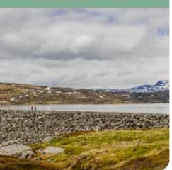
SYSENDAMMEN Is one of Norway's largest stone-filled dams. The total length of the dam is 1.160m, and it consist of 3,6 mill. m3 stone and moraine fell. View of the glacier Hardangerjøkulen from the parking lot.
