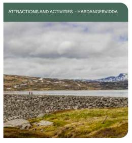
SYSENDAMMEN Is one of Norway's largest stone-filled dams. The total length of the dam is 1.160m, and it consist of 3,6 mill. m3 stone and moraine fell. View of the glacier Hardangerjøkulen from the parking lot.
