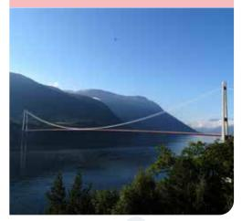
THE HARDANGER BRIDGE opened on August 17th 2013, replacing the ferry connection between Bruravik and Brimnes and reducing the time it takes to drive from Bergen/Voss to Eidfjord. The bridge is a 2 lane suspension bridge with sidewalks for pedestriansand bikers. It is the longest suspension bridge in Norway. The main span is 1310 metres and the total length is 1380 meters, even longer than the Golden
